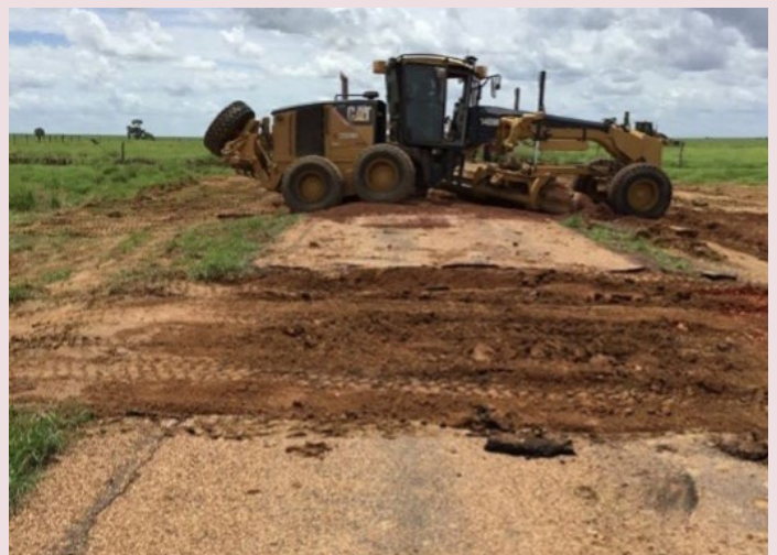
Kennedy Developmental Road (Winton–Boulia) – emergency works
