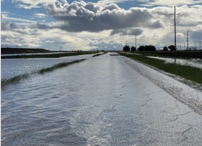
Toowoomba–Cecil Plains Road – flooding from South East Queensland Rainfall and Flooding event (late March 2022)
