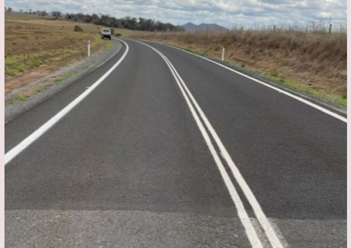
Toowoomba–Cecil Plains Road – completed reconstruction works (November 2023)
