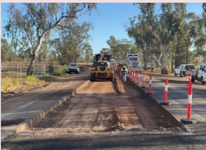
Toowoomba–Cecil Plains Road – reconstruction works (October 2023)
