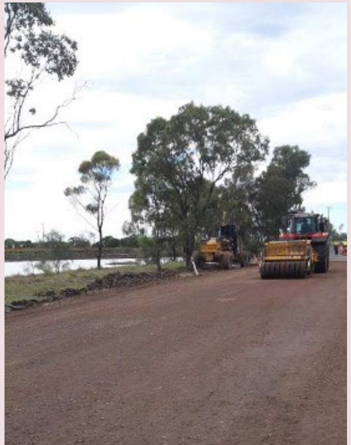
Toowoomba–Cecil Plains Road – emergency works near Condamine River (early March 2022)
