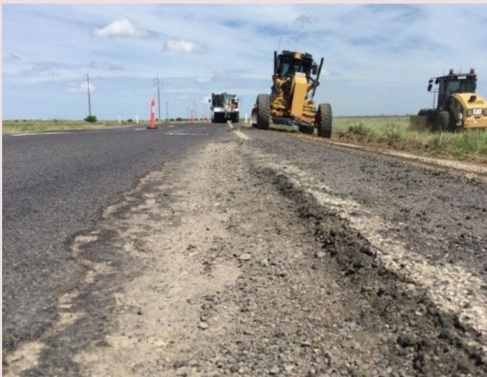
Flinders Highway – emergency works to repair pavement damage
