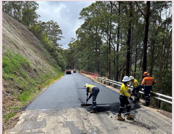
Gold Coast–Springbrook Road – Site 8 repairs (November 2023)
