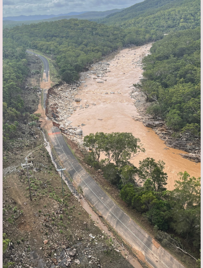
Bloomfield Road in Cook Shire suffered a massive washout as the Bloomfield River became a raging torrent
