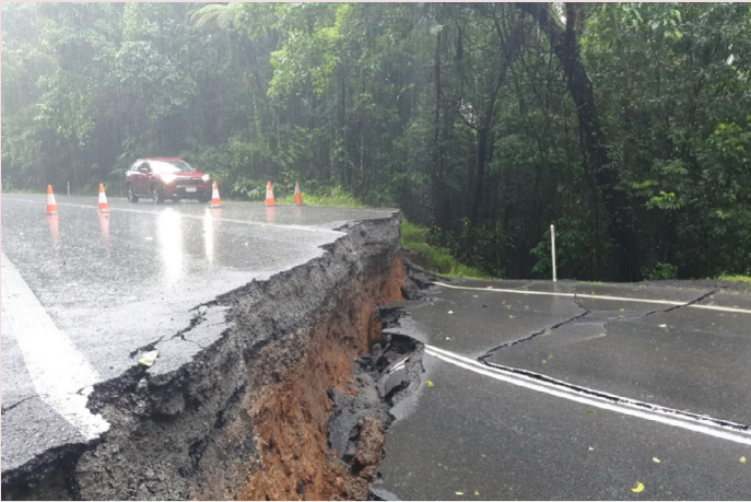
Palmerston Highway – major landslide caused by TC Jasper (December 2023)
