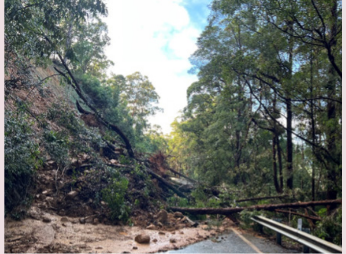
Gold Coast–Springbrook Road – Site 8 landslip following SEQ Rainfall and Flooding event (February 2022)
