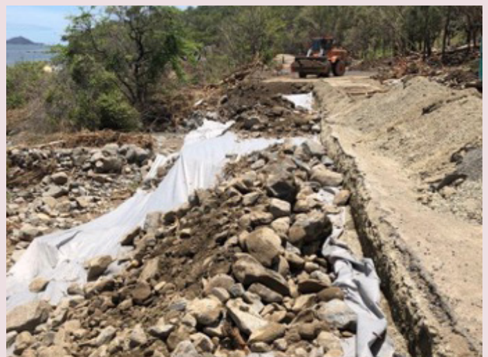
Captain Cook Highway (Cairns–Mossman) – emergency works (December 2023)
