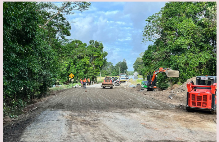
Mossman–Mount Molloy Road – emergency works (December 2023)
