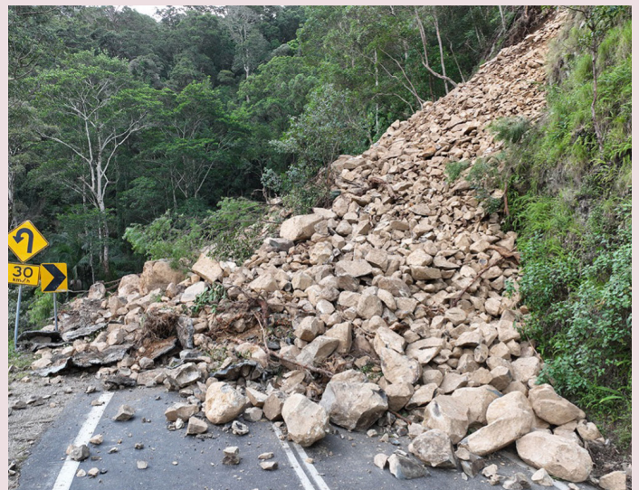
Gold Coast–Springbrook Road – Site 1 landslip (late March 2022)
