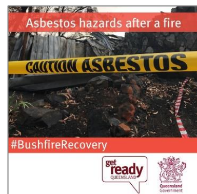
Filename: BushfireRecovery - Asbestos hazards after a fire
