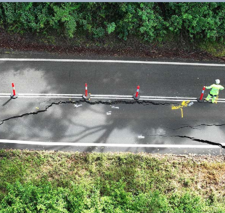
Image top: Beechmont Road – embankment failure (late March 2022). Bottom left: Beechmont Road – embankment failure after SEQ Rainfall and Flooding (early March 2022). Bottom right: Beechmont Road – embankment failure (late March 2022).
