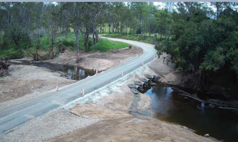
Image: Brooweena–Woolooga Road – repaired Running Creek temporary crossing in February 2022.
