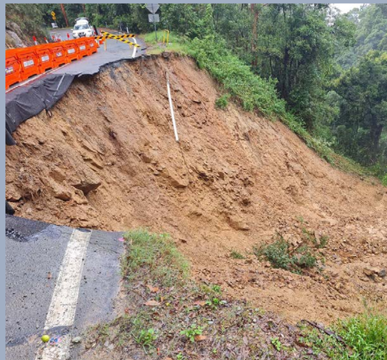
Image top: Beechmont Road – embankment failure (late March 2022). Bottom left: Beechmont Road – embankment failure after SEQ Rainfall and Flooding (early March 2022). Bottom right: Beechmont Road – embankment failure (late March 2022).
