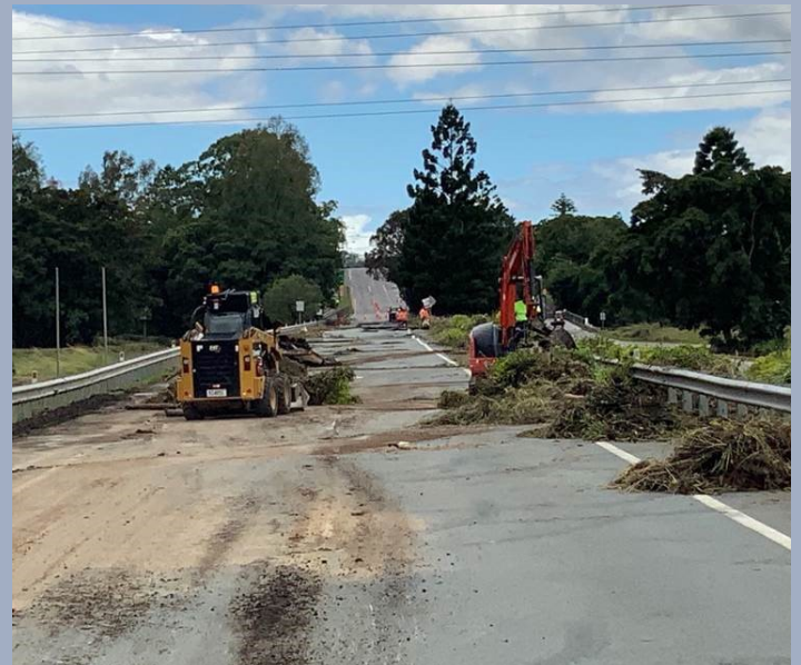
Image: Brisbane–Woodford Road – emergency works in progress.
