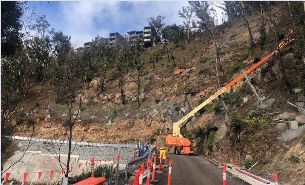
Image: Binna Burra Road – stabilisation works on upslope.
