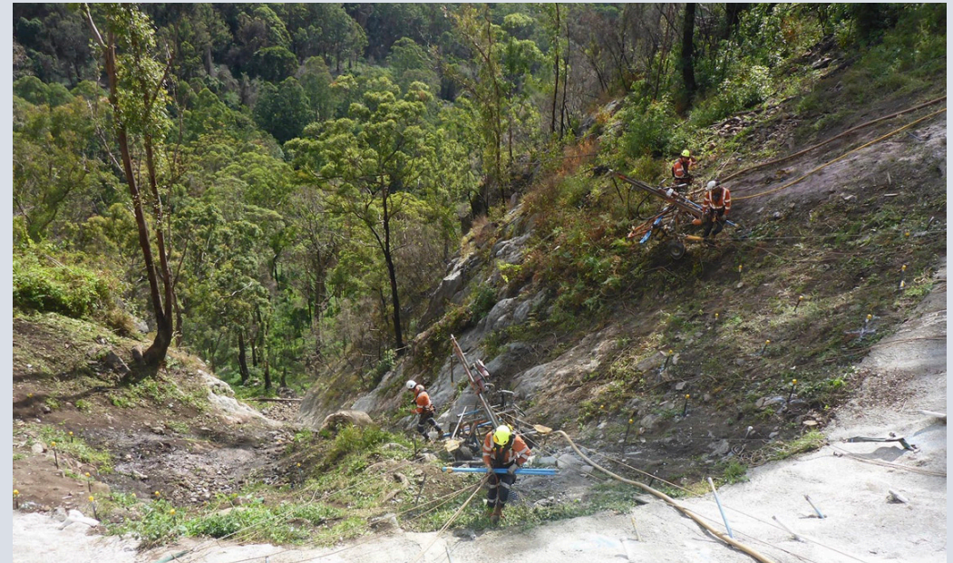
Image: Binna Burra Road – specialist personnel soil-nailing on steep downslope.
