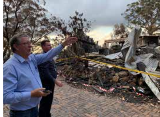
SRC Ian Stewart inspects damage at Binna Burra Lodge
