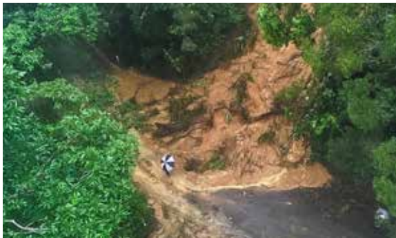
Mount Spec Road – landslip caused by NFNQ Monsoon Trough event
