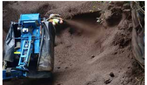
Mount Spec Road – installation of fibrecrete
