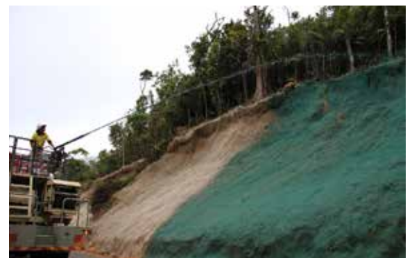
Mount Spec Road – application of hydromulch to assist with revegetation
