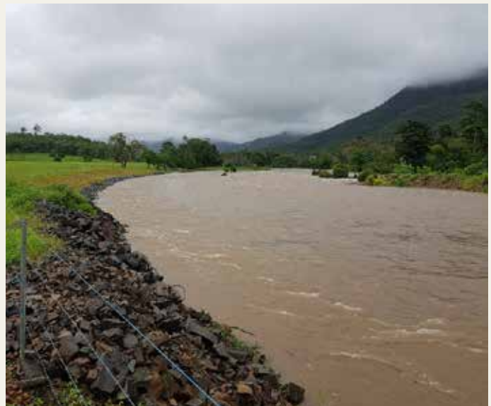
NDRRA works preventing erosion during the Monsoon Event – site SH7 at St Helen’s Creek Source: M. Fahey, landholder
