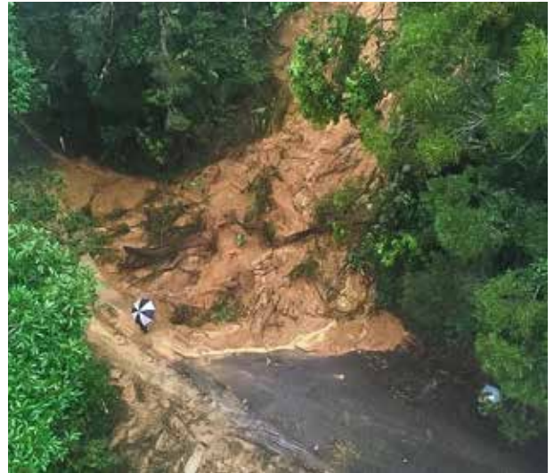
Landslip caused by Monsoon Trough - Mount Spec Road
