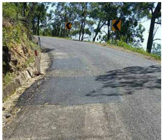
Completed pavement repairs – Mount Spec Road
