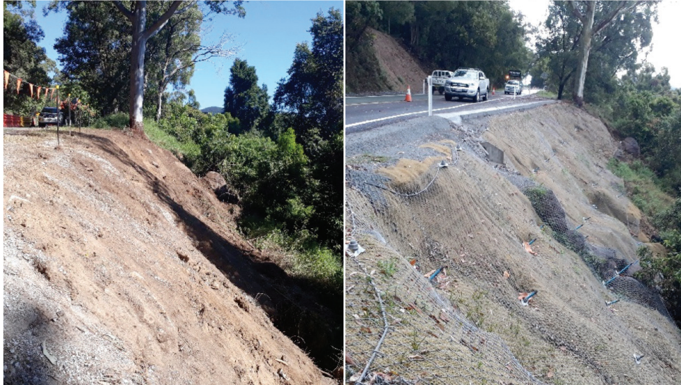
Photos Above: Tomewin Mountain Road – site 6121 damage and completed works
