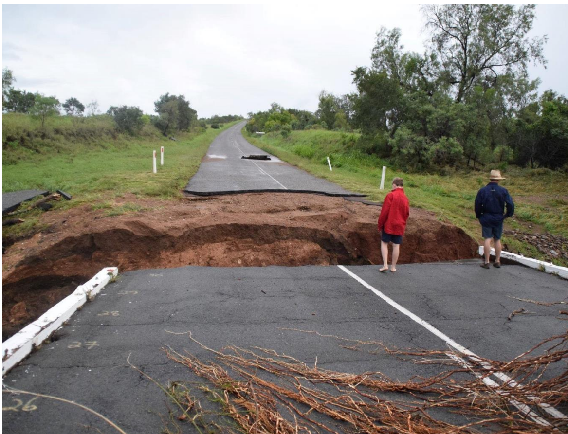
Image: Yatton Creek Bridge, Mackay Regional Council.
