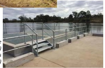
Gayndah Water Intake Station – damage to (above) and post Betterment works (right)
