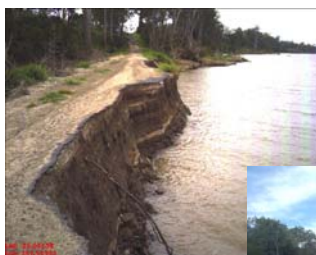
A section of Browns Road washed away following the 2013 floods (above); and the completed realigned road (right)
