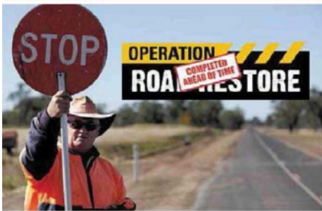
The final works on the Dalby urban road restoration project, Operation Road Restore, were completed in April ahead of schedule and under-budget.
