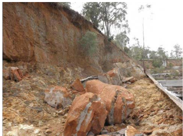
Top: Severe erosion to the banks of the spillway on Gordonbrook Dam
