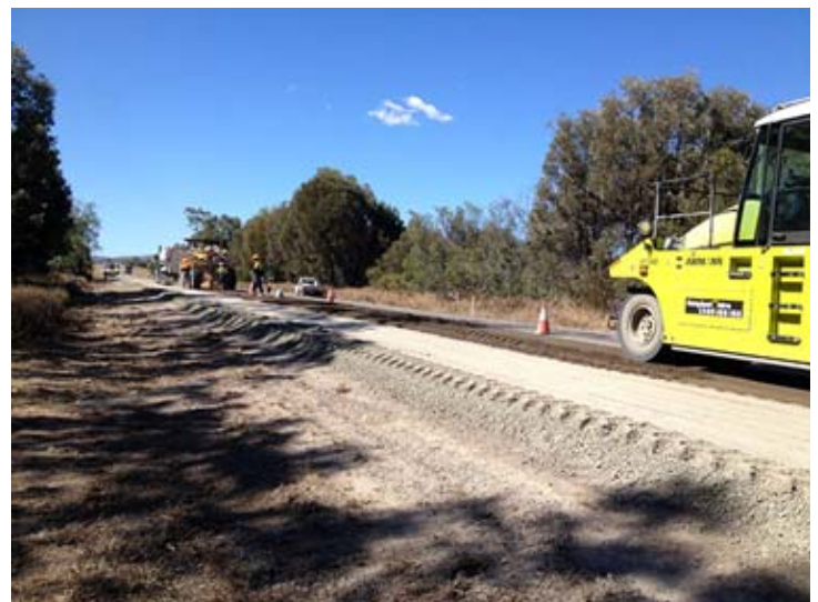
Above: Side track construction on the Warrego Highway.
