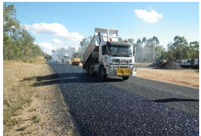
Above: sealing works underway Kennedy Highway, west of Mount Garnet - July 2014
