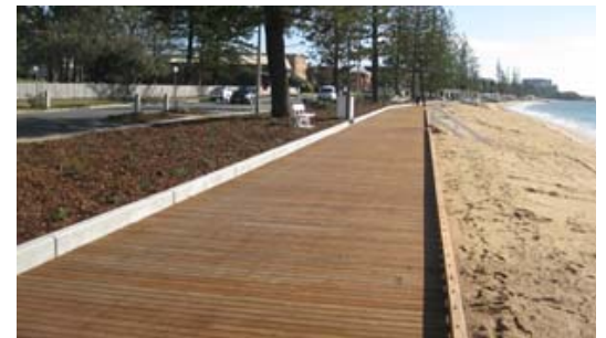
Damage to (top) and following betterment works on Margate seawall project - August 2014 (bottom)
