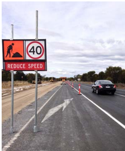
Left: Pavement stabilisation works on the Dawson Highway
