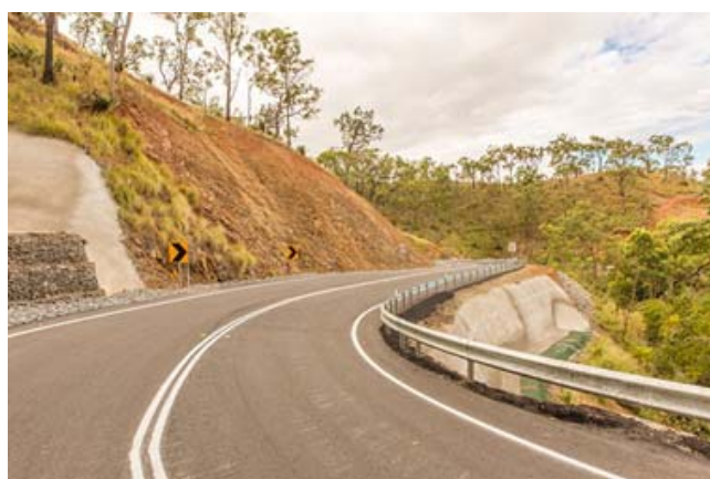
Top: Landslips and damage to the Mount Morgan Range following Tropical Cyclone Oswald
