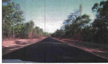
The sealed road after the works were completed
