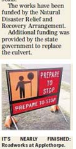
IT'S NEARLY FINISHED: Roadworks at Applethorpe. PHOTO: FILE
