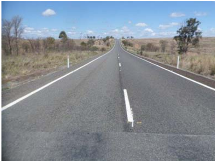
Above: Completed works on the Dawson Highway
