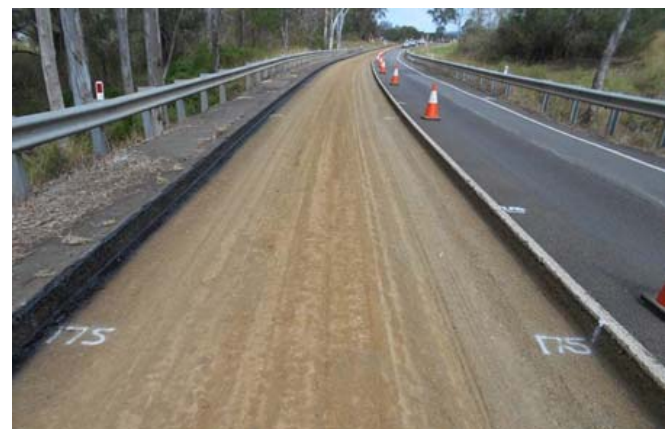
Above: Rosewood–Warrill View Road – preparation for asphalt works
