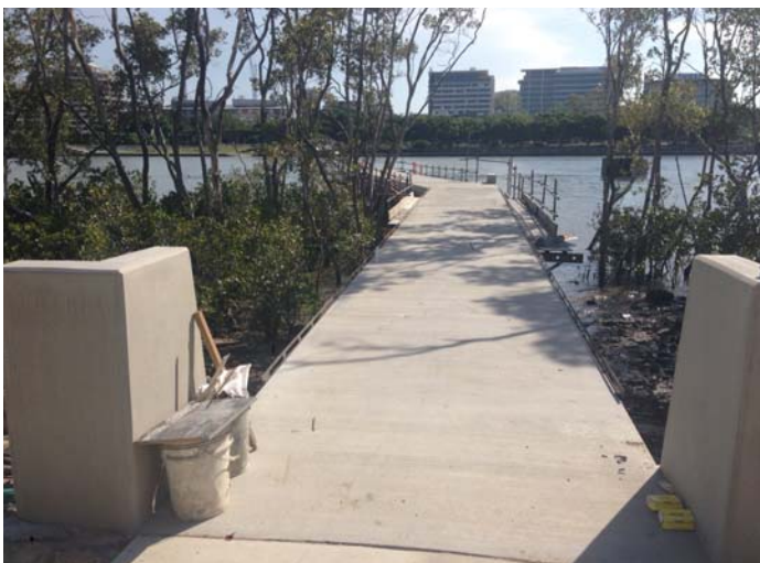
Left: Progress of construction on QUT Gardens Point ferry terminal - October/November 2014
