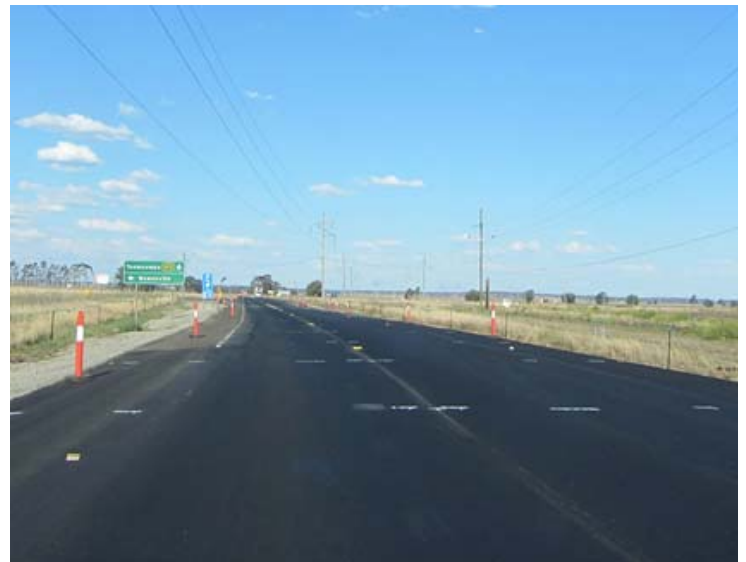
Right: Warrego Highway works at Bowenville.
