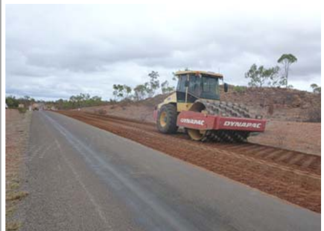
Above: grave compaction works underway on the Cloncurry to Dajarra Road - March 2014
