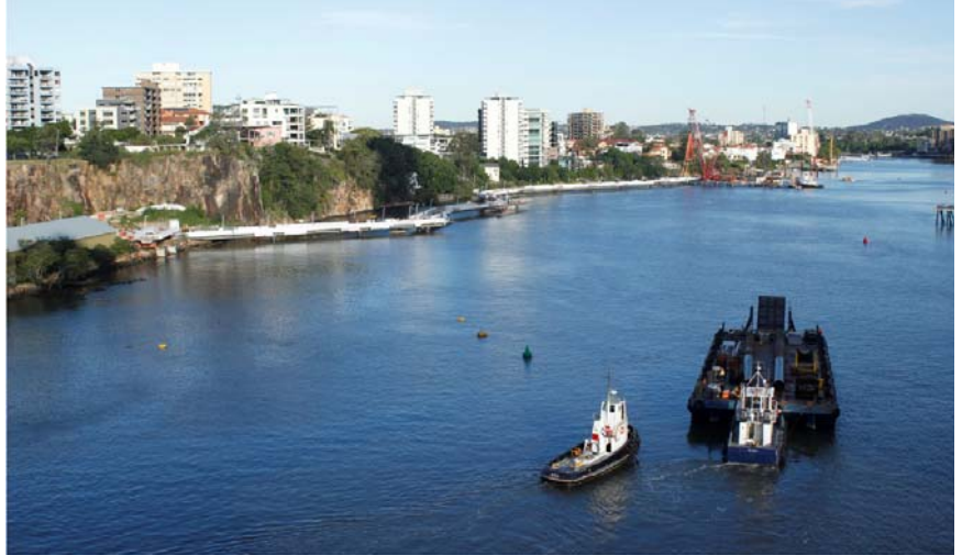
Steel liners being transported to site whilst the 16th girder is lowered onto the pier searing plates
