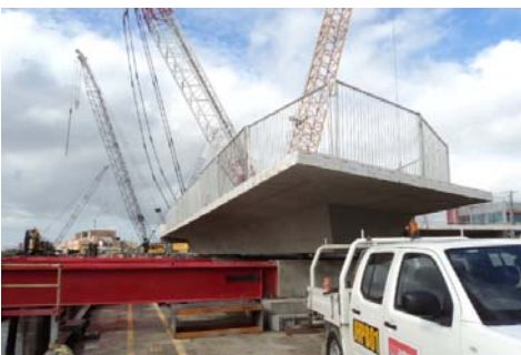
Electrical cables being fitted to the underside of a girder (top) and girder being lifted onto the load out facility for the barge (centre and bottom)
