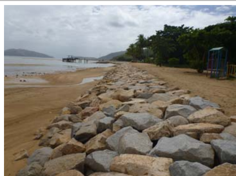
Works underway to Palm Island Seawall, May 2014, showing completed rockwall (left) and concrete section under construction (centre and right)
