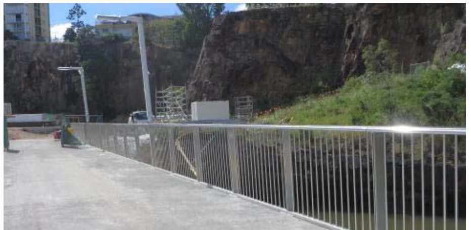
Right: the new Riverwalk balustrade
