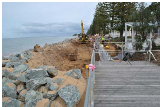
Works underway on Margate Seawall - May 2014
