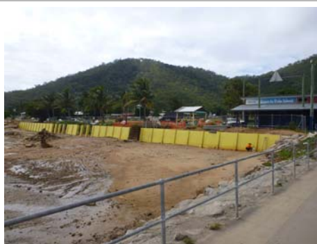
Works underway to Palm Island Seawall, May 2014, showing completed rockwall (left) and concrete section under construction (centre and right)
