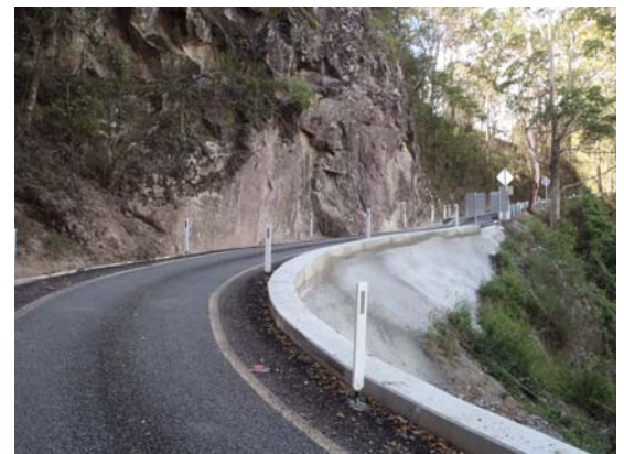
Following reconstruction works (inclusive of complementary works) on Grigor Bridge (top) and Ob-Obi Road (bottom)
