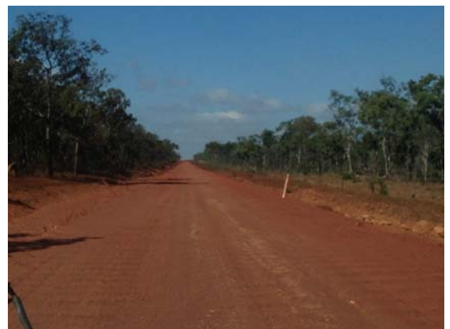
Right: Damage to (top and centre) and following reconstruction works (bottom) to Bamaga Road
