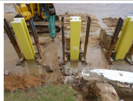
Works underway to Palm Island Seawall, May 2014, showing completed rockwall (left) and concrete section under construction (centre and right)
