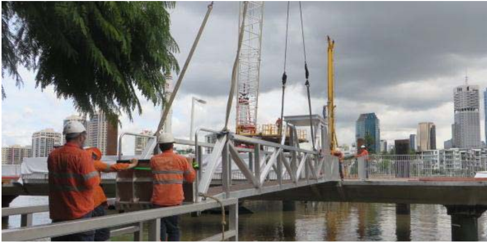
Above: gangways being installed
