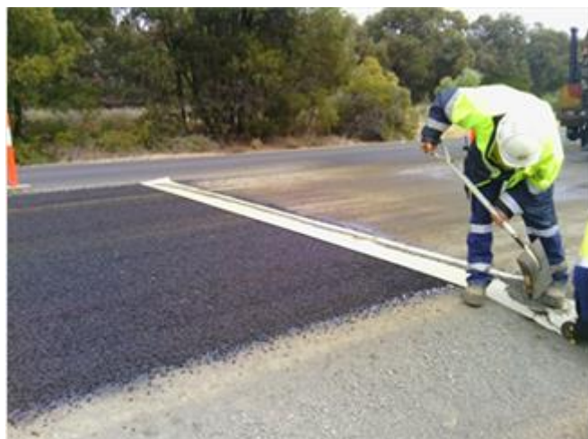
Above: Warrego Highway – sealing work between Dalby and Miles
