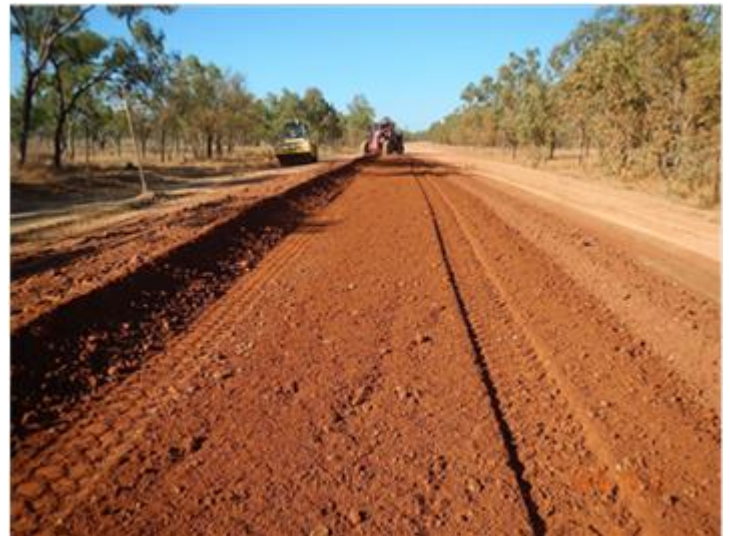
Burke Developmental Road – grading in progress
