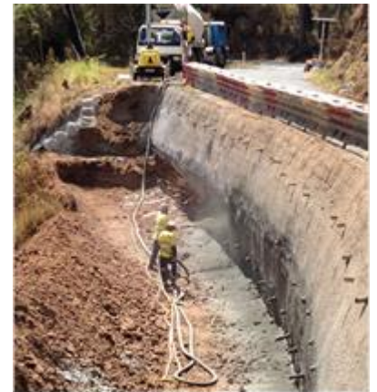
Shotcreting the batter after the installation
