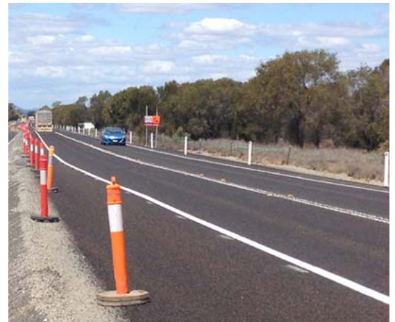
Warrego Highway works - traffic switched onto newly reconstructed section at Jondaryan.
