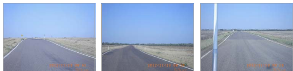
Above: showing restoration of sections of Cannington Road.
