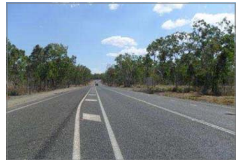
Above: Peak Downs Highway – completed section.
