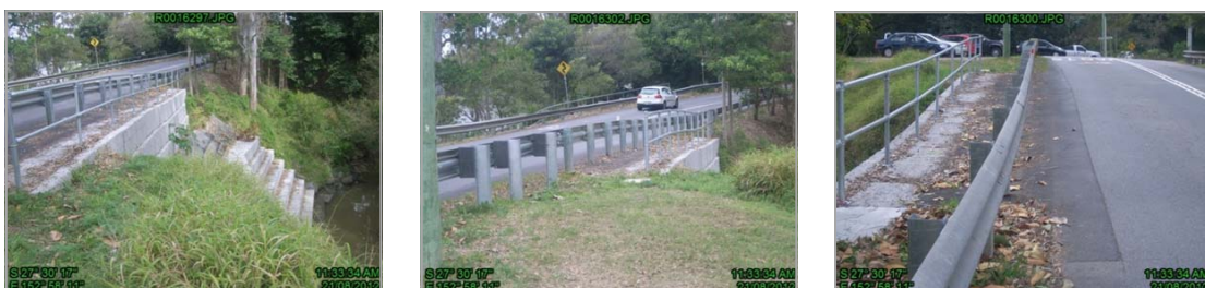
Above: completed block retaining wall for embankment protection along Radnor Street.
