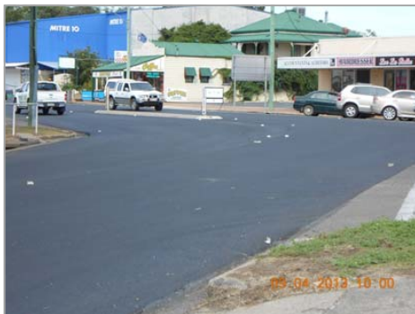
Above: Works prior to linemarking in Millmerran.
