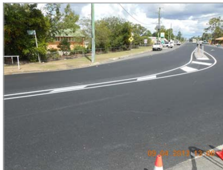
Above: Completed linemarking in Millmerran.
