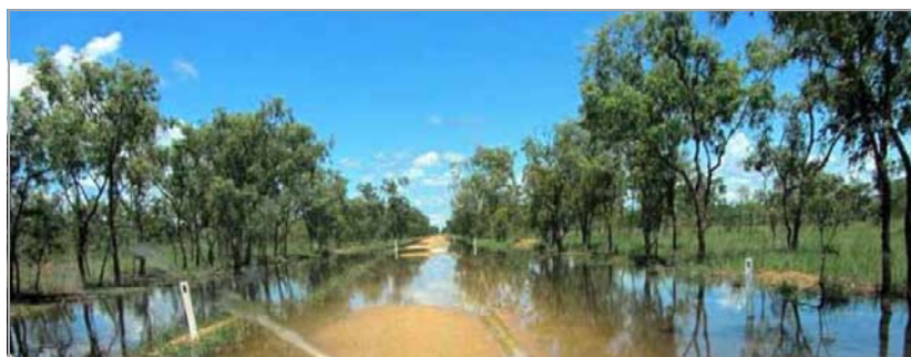
Above: Flooded Burke Development Road - 19 February 2013 (Image courtesy TMR)
