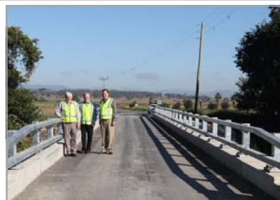
From left Cr Duncan McInnes, Scenic Rim Regional Council's Patrick Murphy and Mayor John Brent inspect the newly completed Stokes Bridge at Silverdale.
