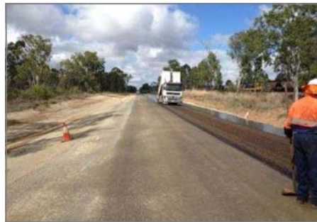
Above: Primer sealing on a section of the highway.
