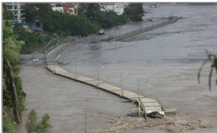
Above: damage to Brisbane RiverWalk during January 2011 floods.
