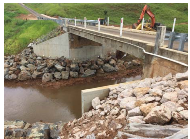
Right: Seamark Road Bridge pictured before reconstruction, during project works
