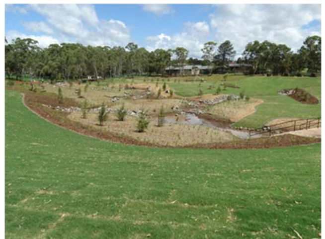
July 2015 - Garnet Lehmann detention basin following flood mitigation works
