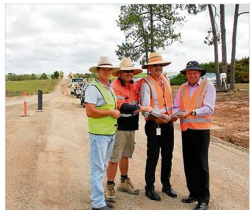
ARE WE THERE YET? Primary Production and Rural Infrastructure Portfolio Councillor James Hansen, JAC Civil site supervisor Simone Betts, Fraser Coast Regional Council Executive Manager Works and Services Bryan Hart and Infrastructure and Planning Portfolio Councillor Trevor McDonald check progress on Yerra Rd. PHOTO: CONTRIBUTED
