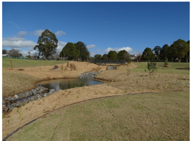
July 2015 - Ballin Drive detention basin following flood mitigation works
