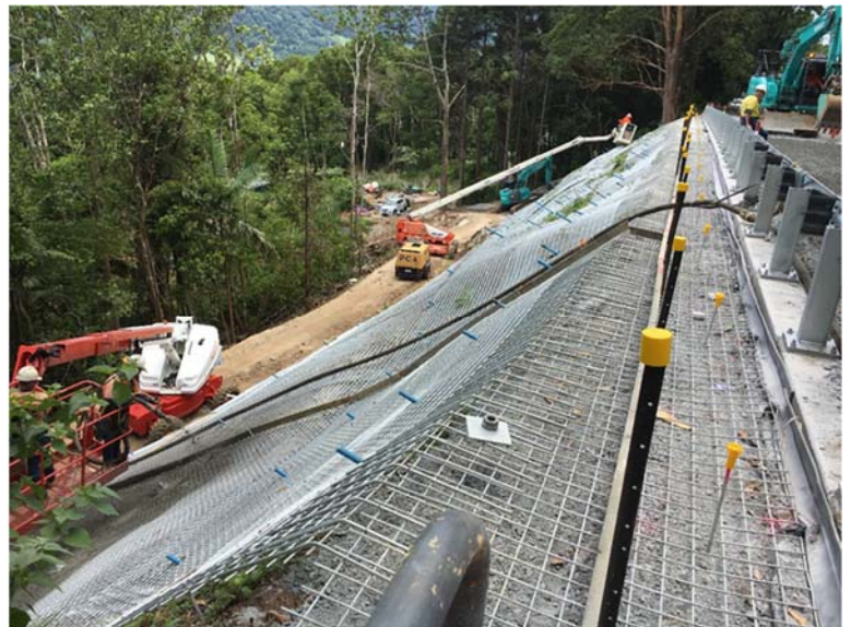
Reconstruction works at main landslip site on Tomewin Mountain Road
