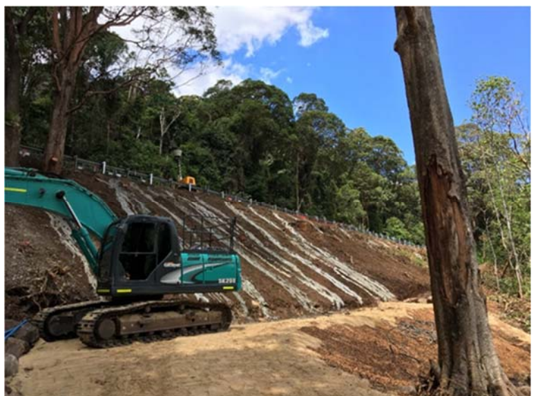
Site preparation at Tomewin Mountain Road
