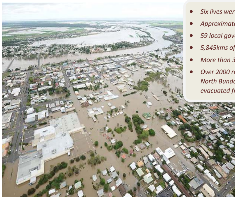
Aerial photo of Bundaberg following TC Oswald, showing the extent of flooding
