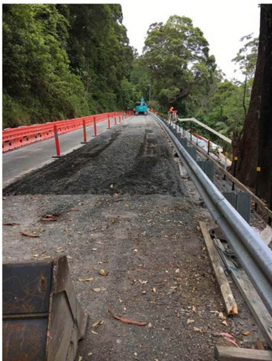
Reconstruction works at main landslip site on Tomewin Mountain Road
