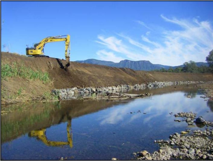
Work underway reconstructing the left bank of Warrill Creek, Scenic Rim
