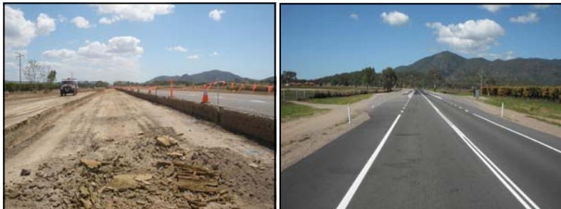
Works in Progress October 2011
